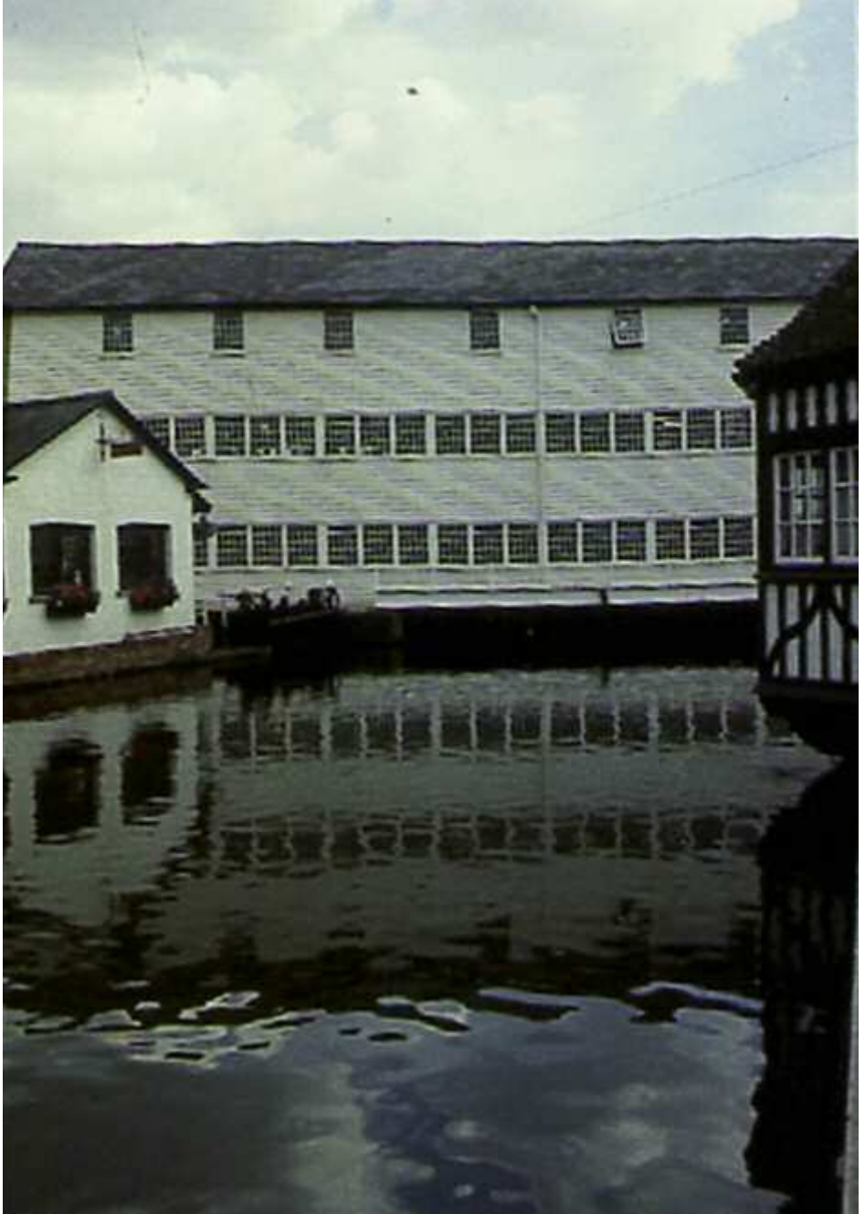
Functional timber buildings, exemplified by Courtauld's 18th-century weaving sheds at Halstead, Essex, pointed ahead to further structural innovation, particularly in naval dockyards.
