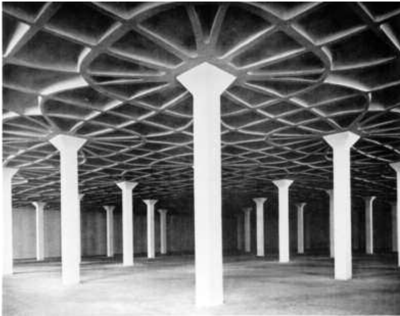
Concrete vaulting and columns for the Gatti Wool Mill, Rome, 1951, engineer Pier Luigi Nervi. Elsewhere Nervi mastered spanning of large expanses with reinforced concrete, for hangars, sports stadia and exhibition halls.
