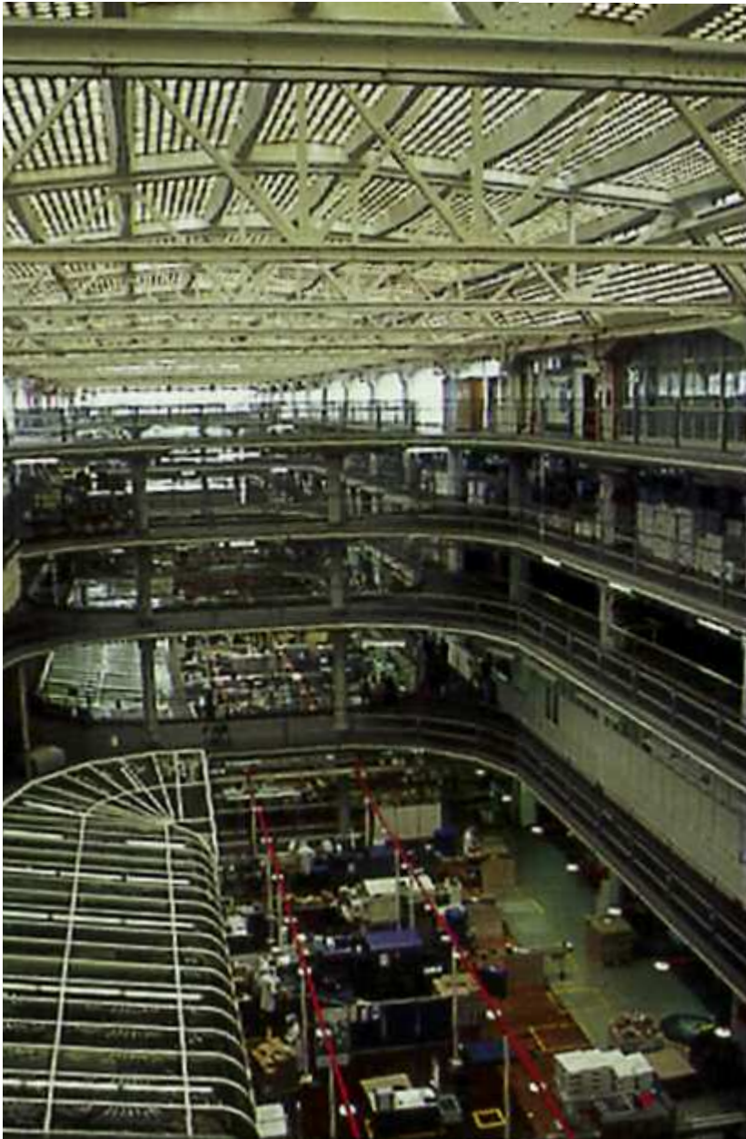
The packing hall at Boots' 'Wets' factory, seen in 2001. The shutes have gone and an enclosed ground-floor area has been added, bottom left, but there are few other major changes, 70 years on.
