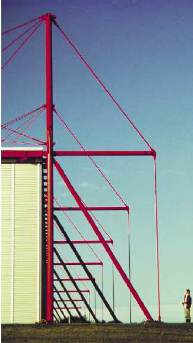
Masts and steel bracing rods around the building denoted new technology at the American-owned Fleetguard Manufacturing & Distribution Centre, Quimper, Brittany, 1979–81, architects Richard Rogers Partnership.
