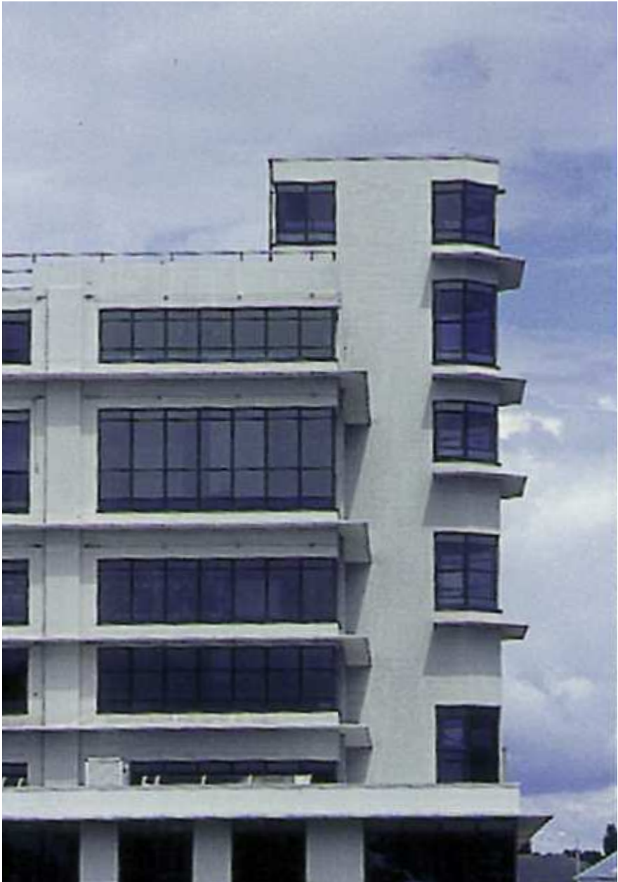
Boots' 'Drys' factory, Beeston, 1937–8. Owen Williams's second building on the site was a more conventional structure due, in part, to the change of ownership from American to British.
